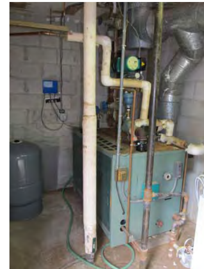
Central boiler for production of hydronic heat at Building 1 is nearing the end of its expected useful service life
