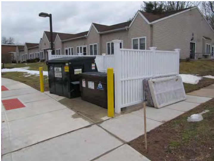
Recently installed dumpster enclosure is constructed of vinyl stockade fencing
