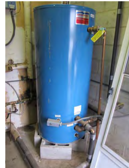
Typical (one of two) domestic hot water storage tanks at Building 2
