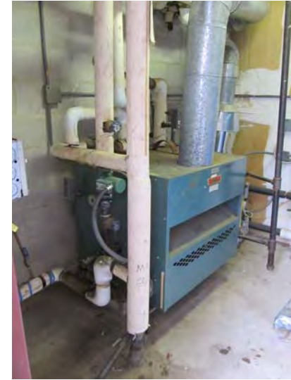
One of two boilers for production of hydronic heat at Building 2
