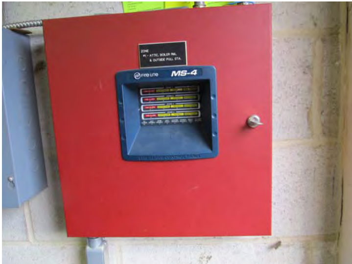
Original zone-type fire alarm control panels typical at both buildings
