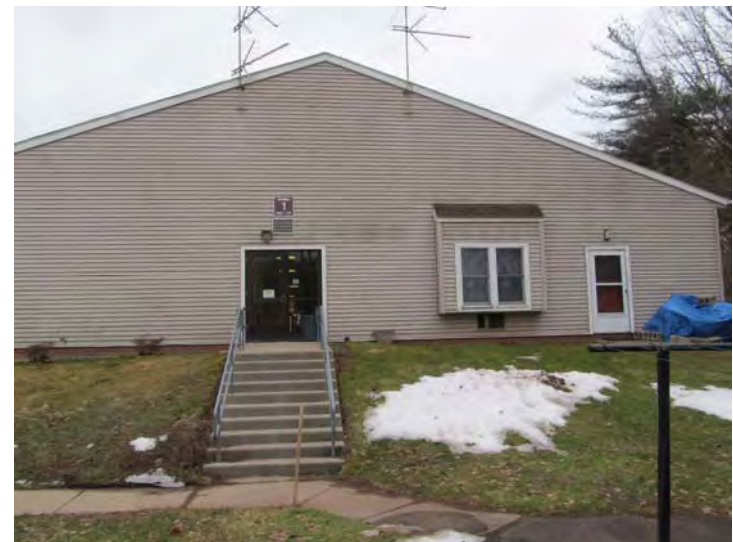
Original vinyl siding is in good overall condition
