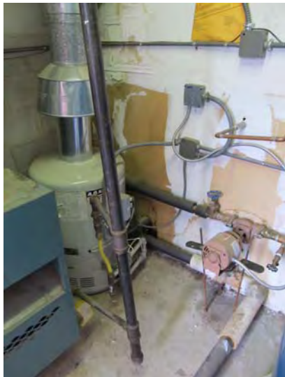
One of two boilers for production of domestic hot water at Building 2
