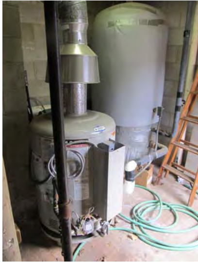
Boiler and storage tank serving domestic hot water system at Building 1
