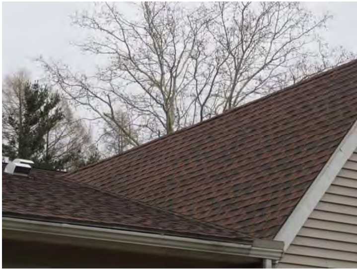
Newer architectural-style shingles typical on roof surfaces at both buildings – No problems noted
